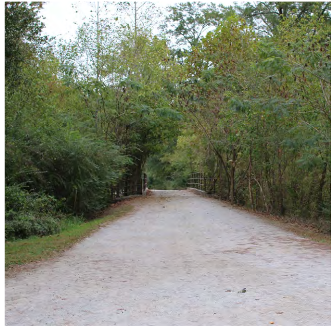
Figure 3: Crushed aggregate trail at Cochran Shoals Trail
