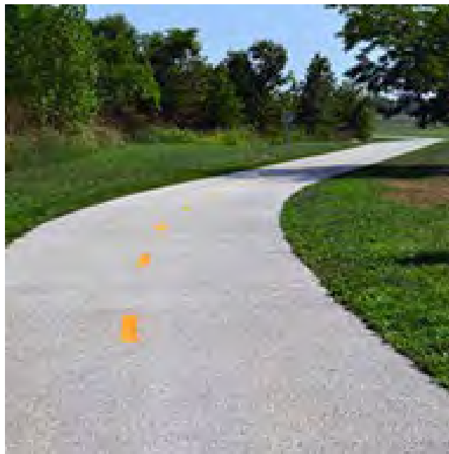
Figure 9: Pervious concrete bike path
