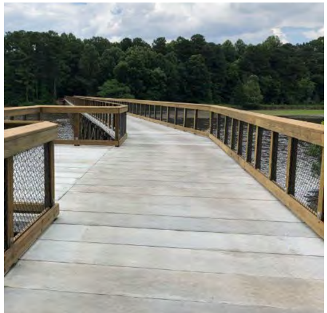
Figure 6: Reinforced, precast concrete panel boardwalk from PermaTrak
