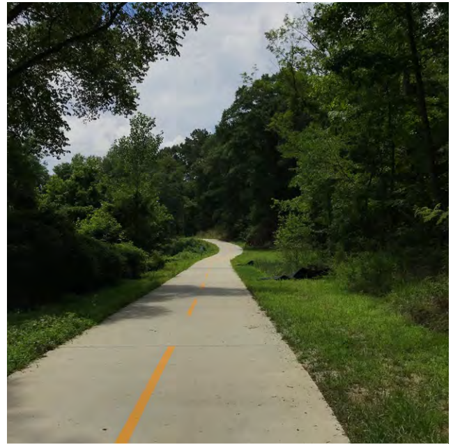
Figure 1: Concrete Trail at the Proctor Creek Greenway
