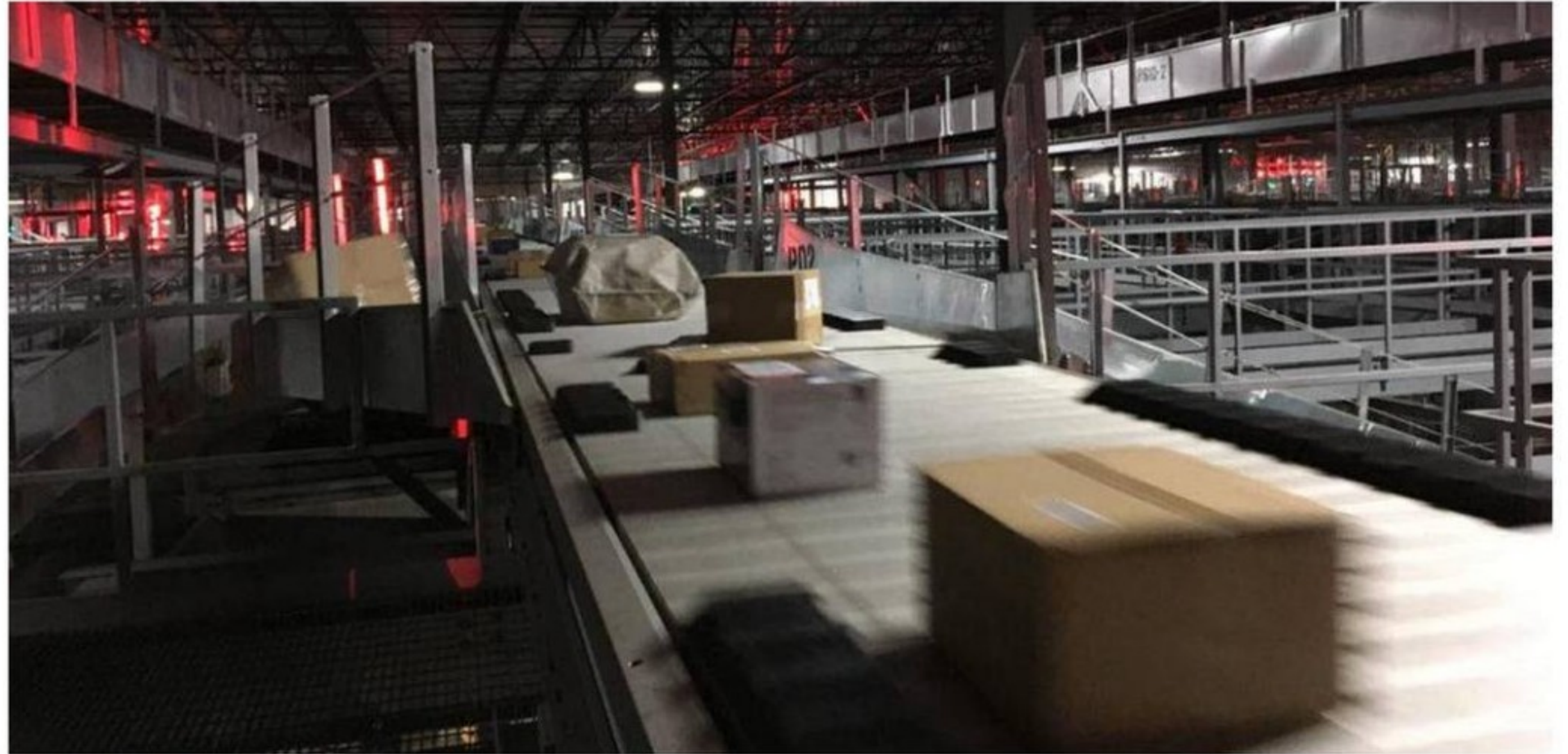
UPS SMART Hub
